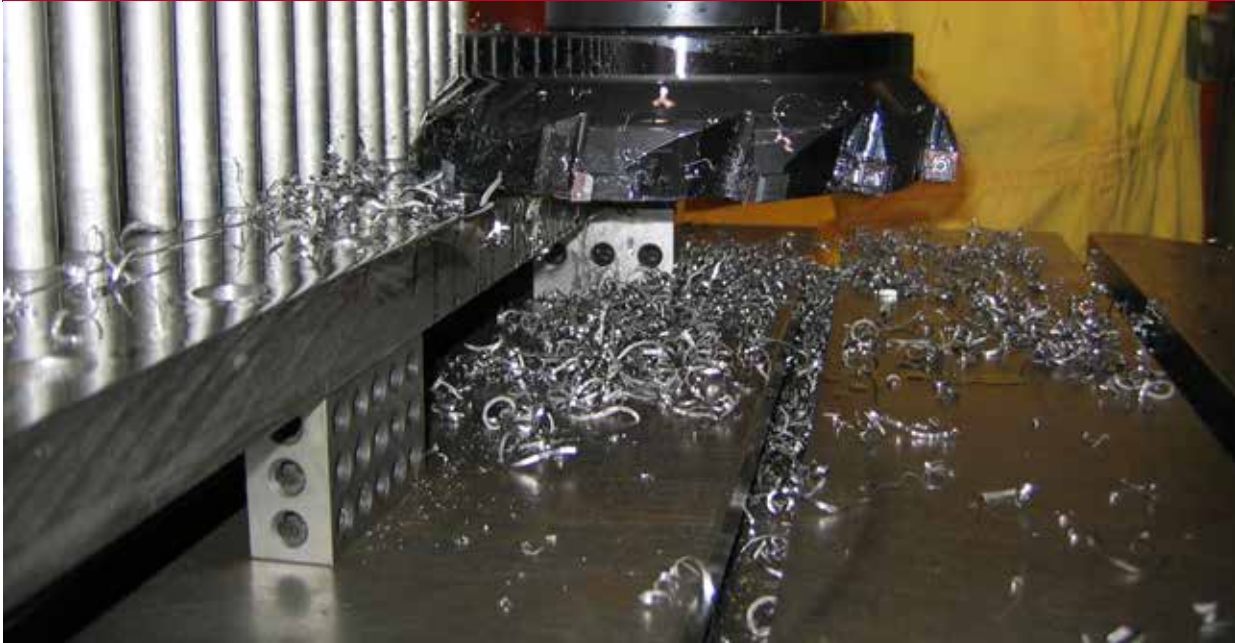
Restoring a Heat Exchanger Gasket Surface
