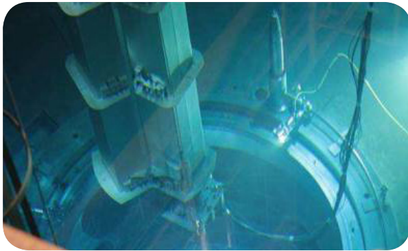
Core data acquisition (same number of high-resolution pictures as number of fuel assemblies)
