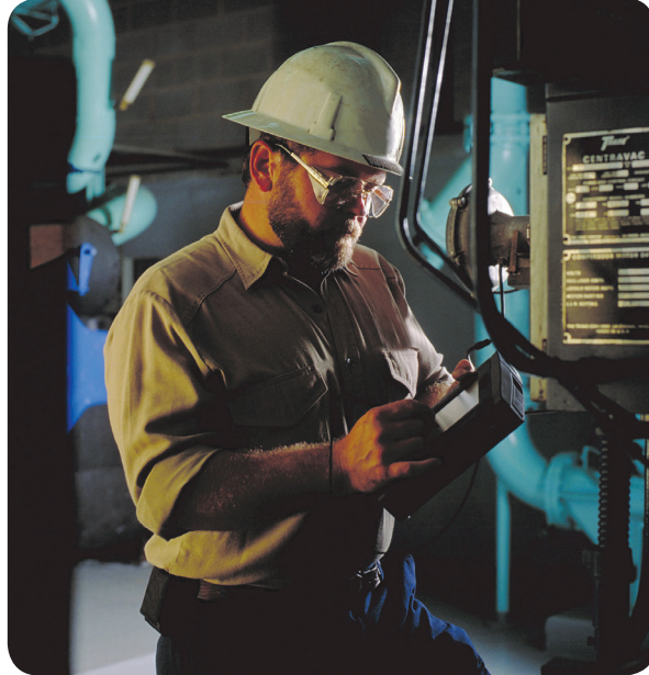
Vibration surveys utilize microprocessor-based computer systems, which provide a fingerprint of the operating condition of machinery.
